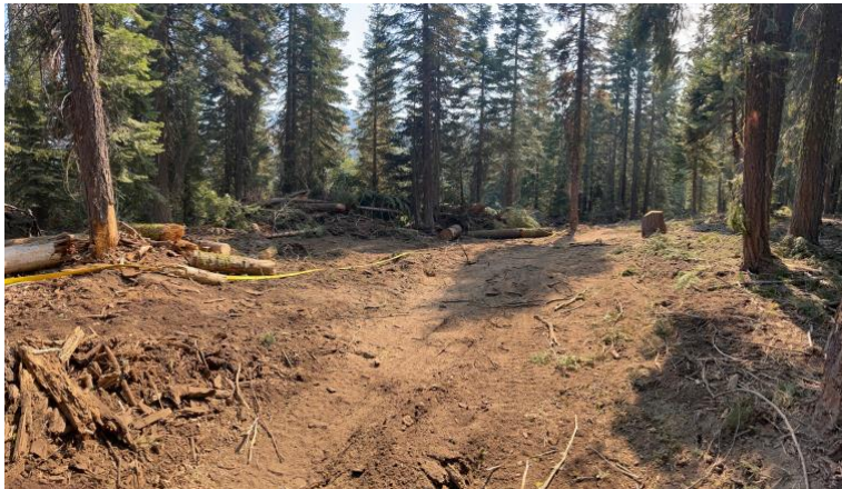
The Boulder Lake Trail leading into the Trinity Alps Wilderness was bulldozed by fire crews during suppression of the River Complex Fire. Photo credit: Amanda Barragar
